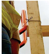
PHOTO COURTESY OF KIEWIT POWER CONSTRUCTORS
